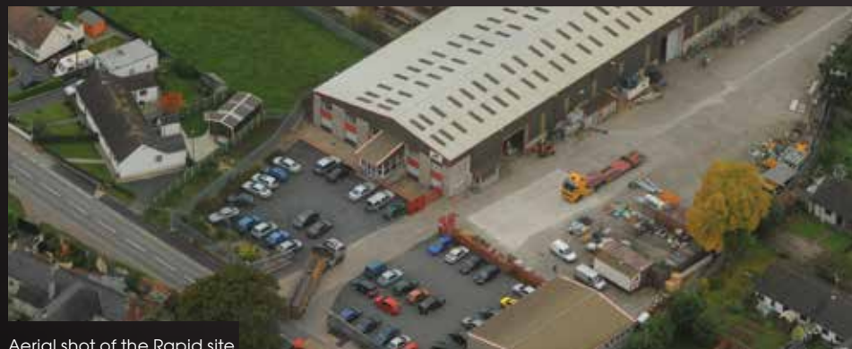
Aerial shot of the Rapid site
