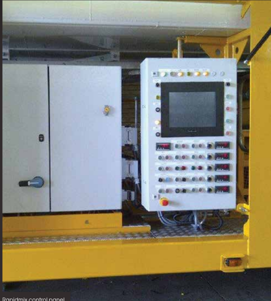
Rapidmix control panel
