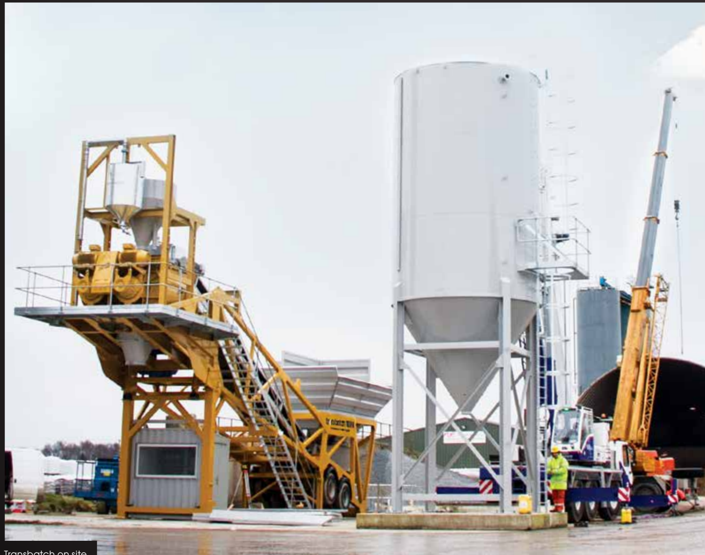
Transbatch on site
