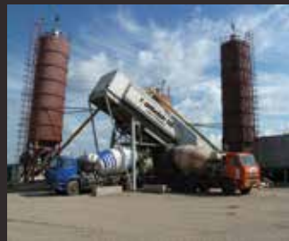
Concrete road building and readymix Russia
